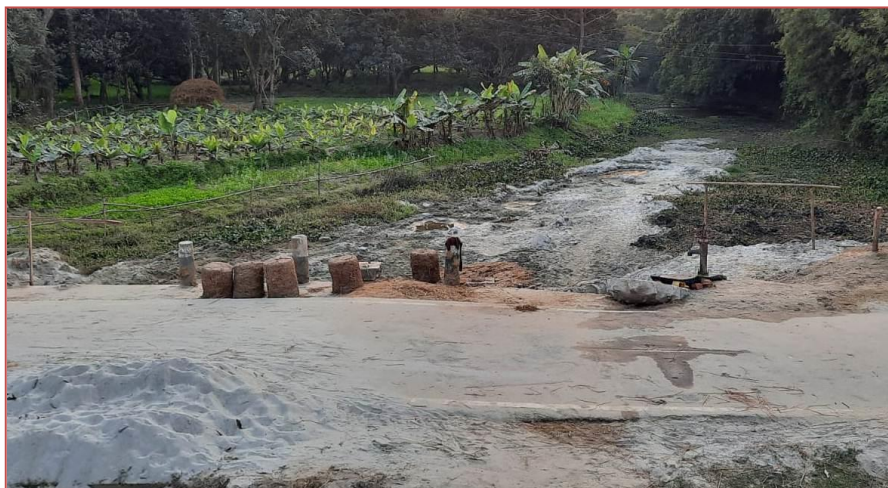
Fig.8 Loss of flow in canals due to heavy sand deposits, a common feature in canal networks in the district.
